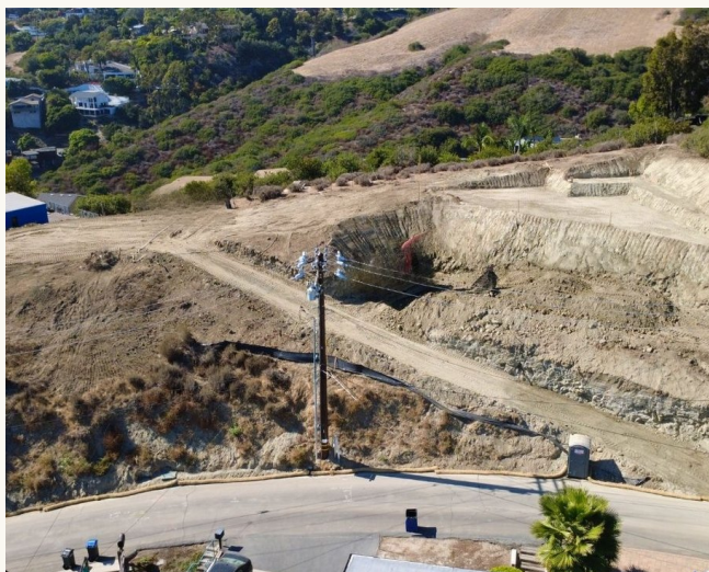
The excavated, benched building pad at 1560, and a straight-down aerial of the graded lot.
